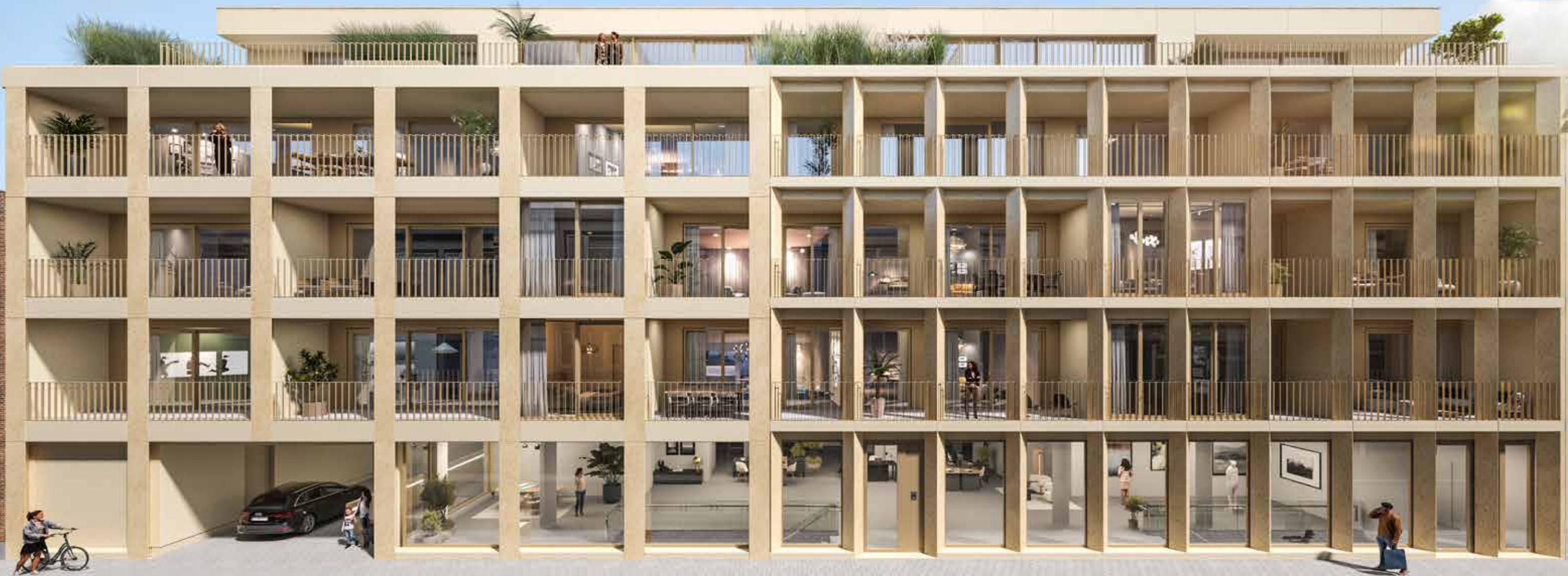
The Vault, Antwerpen — Van Wellen Real Estate Development
